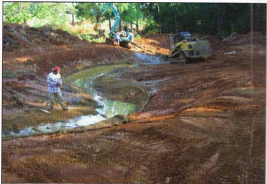
Restoration of White Creek meant re-creating the rural streams natural meandering type of channel (above) and adding pools, boulders and other features for fish habitat while installing natural fiber products, like coir erosion control blankets, to stabilize the streambanks (below).
