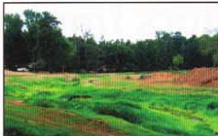
Not long after construction was completed, this stand of grass is helping to control erosion.
